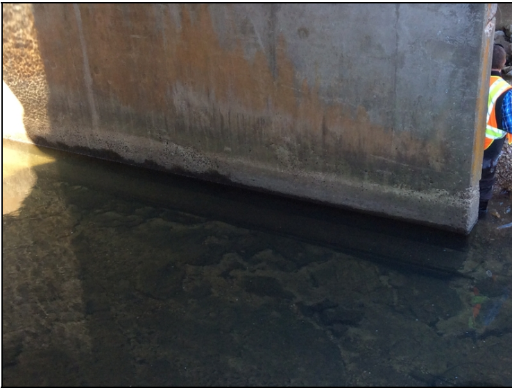
Scour up to 1' below top of footing @ Bent 2.
