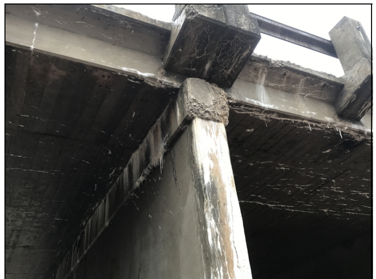
Deterioration & efflorescent map cracking to Left & Right ends of Cap @ Bents 1 - 5.
