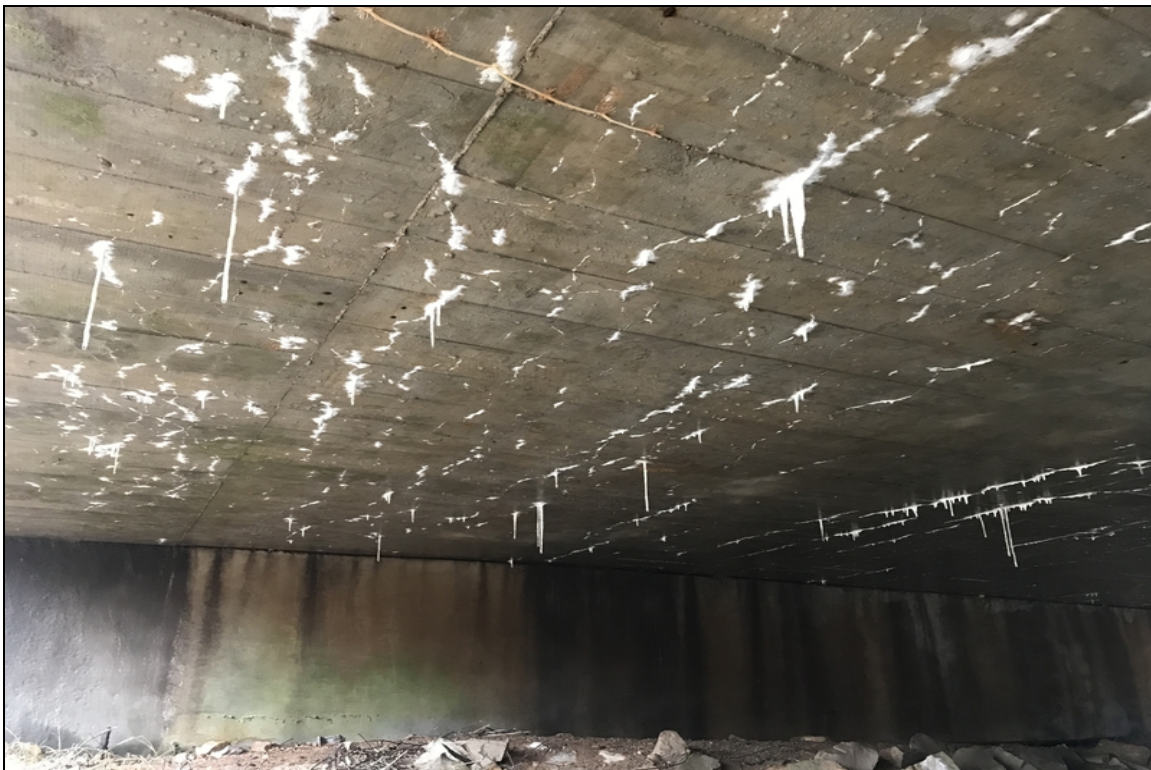
Typical efflor cracksnto soffit @ all spans.
