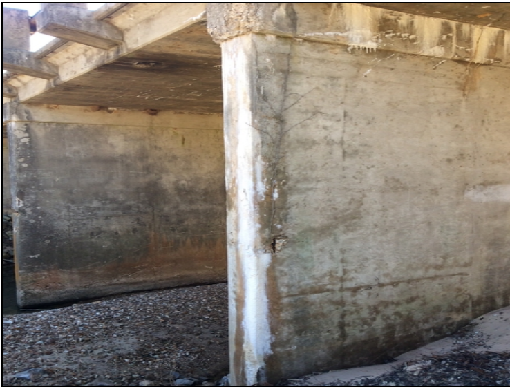
Spalls/delaminating with efflorescence, Rebar & wire mesh exposed to Pier walls @ Bent 3.
