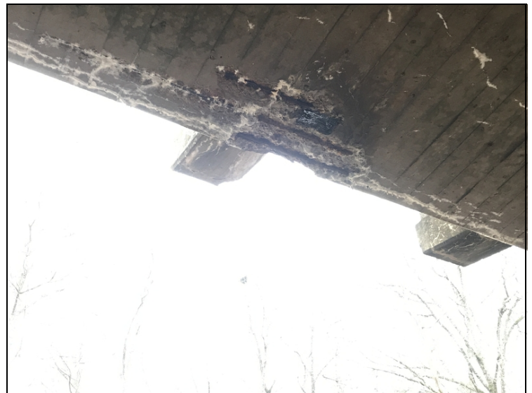
Spalls with Rebar Exposed to Deck below @ Spans 4 & 5.
