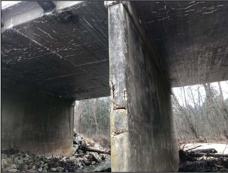
Spalls/delaminating with efflorescence, Rebar & wire mesh exposed to Pier walls @ Bent 2 & 3.
