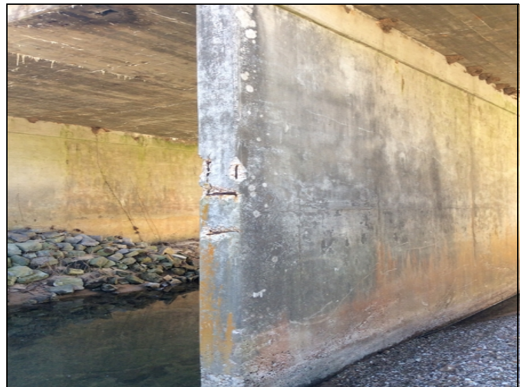
Spalls/delaminating with efflorescence, Rebar & wire mesh exposed to Pier walls @ Bent 2.
