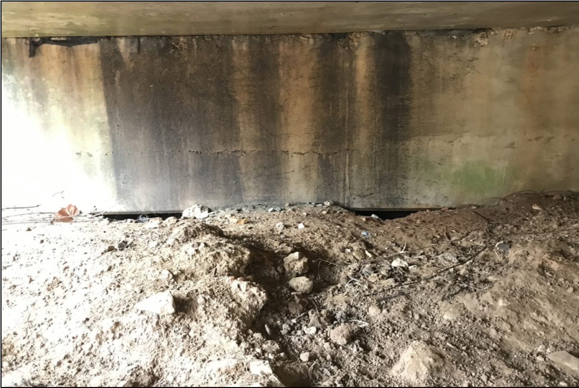
Minor settlement to abutment 2.
