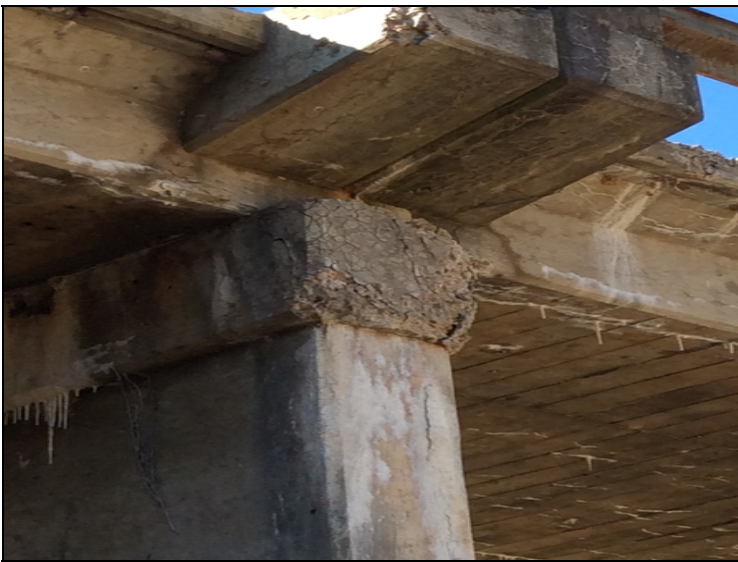
Deterioration & efflorescent map cracking to Left & Right ends of Cap @ Bents 1 - 5.
